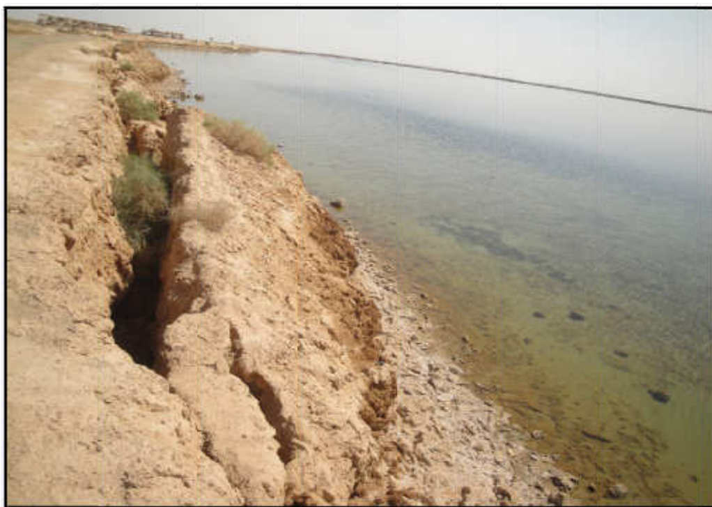
Figure 5-17: The collapse of the lake wall due to chemical dissolving causing increase the surface area of the lake.
